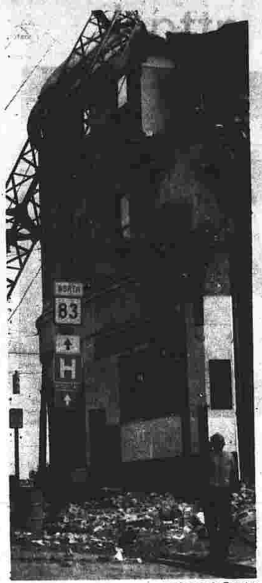
Demolition continues ... slowly and stubbornly
